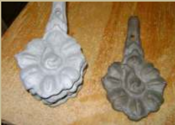
Photo, left: Missing decorative elements can be recreated by using existing elements and creating a cast.
