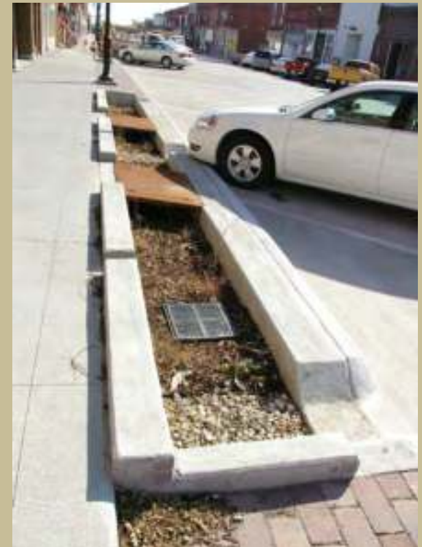
Photo, above: A sustainable rainwater runoff system was carefully designed into this historic district’s new street in a way that did not detract from the historic qualities of the district.
